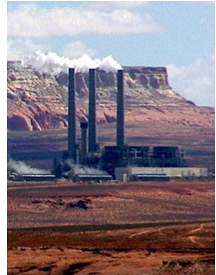
Navajo Power Plant
