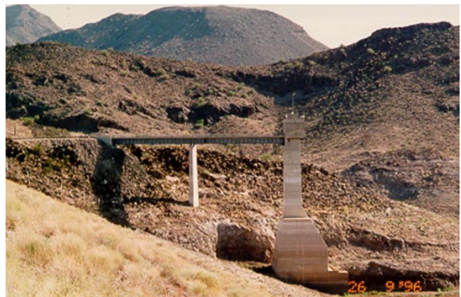
Painted Rock Control Tower, photo credit: USACE
